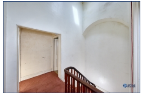
Third Floor Staircase
