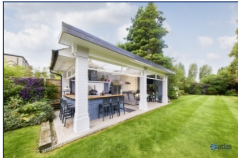
Summer House/Patio/Dining Area
